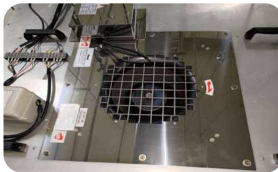
Hsinchu Plant replaced energy-efficient DC FFU.
