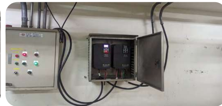
Toufen Plant Installed a 20HP variable frequency drives on Condensate Pump
